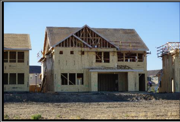
Neighborhood C – Under Construction
