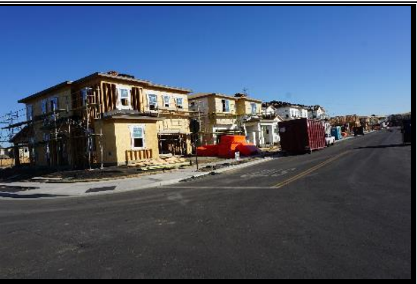
Under Construction Neighborhood D
